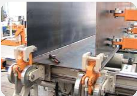
WELDING OF BOX SECTION
